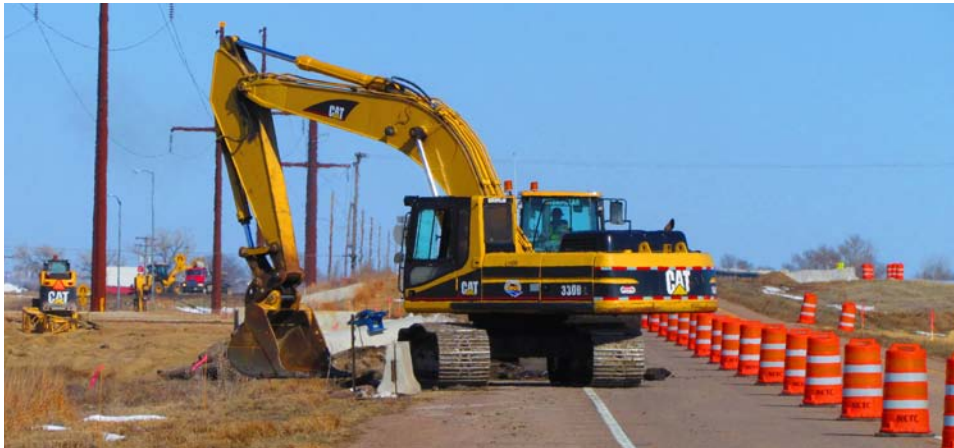
Highway construction cone zone on I-76
